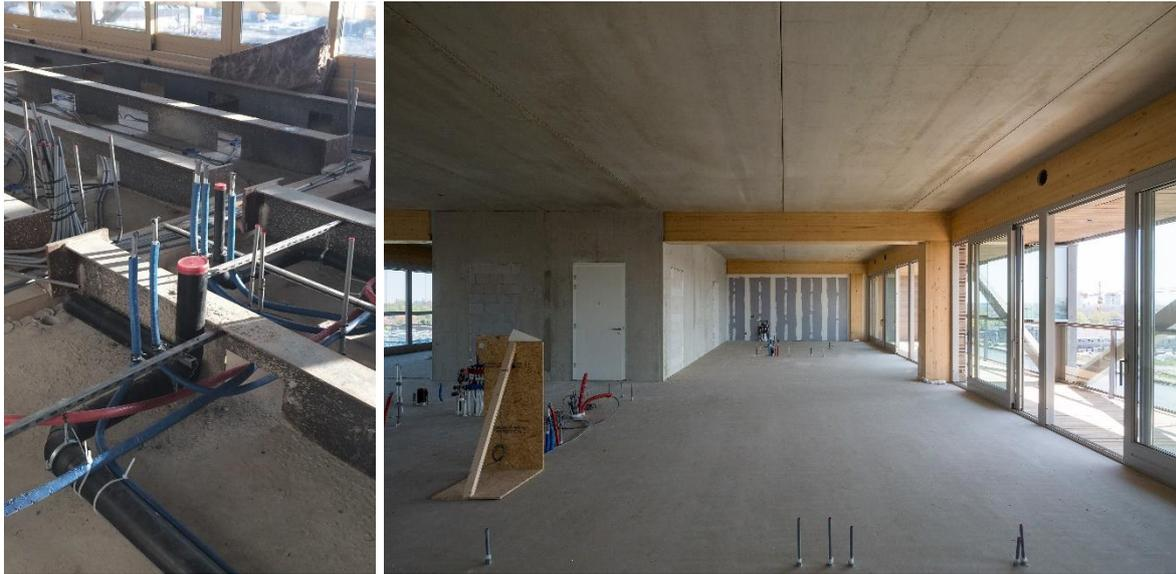
Figure 5: The hollow floor giving access to hollow space with pipes and cables as constructed, without the top floor.
