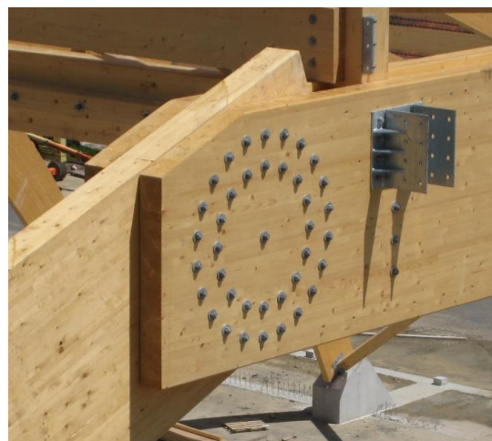
Figure 9 : Liaison arc-traverse
