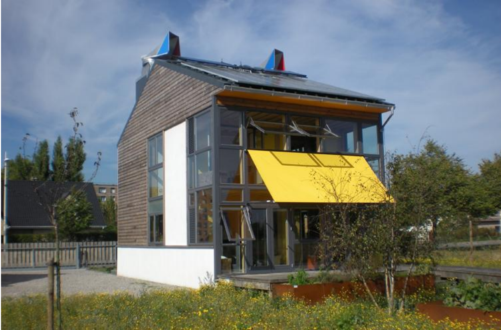
Image 2: maison RuralZED – Agence ZEDfactory
